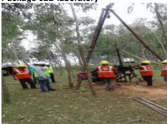
Geo-technical Investigation at Borehol-1 Pedda OHSR site Package-02B
