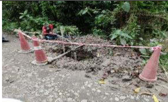
Barricading with caution tape at hydro testing process seen at zone-4(Pipe line site)
