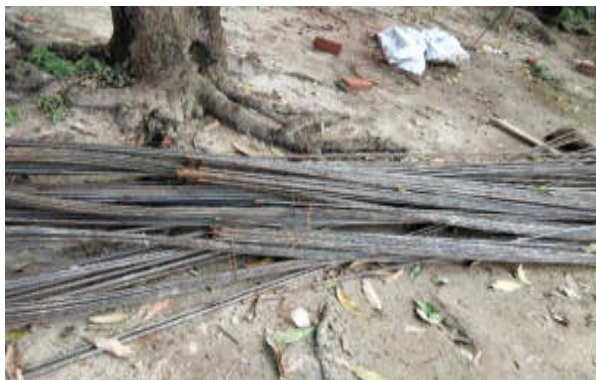
Poor storage condition of reinforcement bar at construction site
