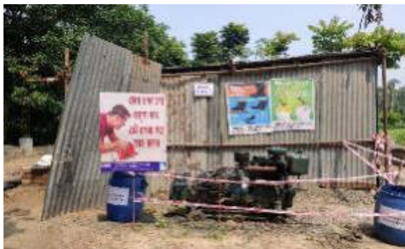
Diesel generator at zone-4(OHR) without spill containment
