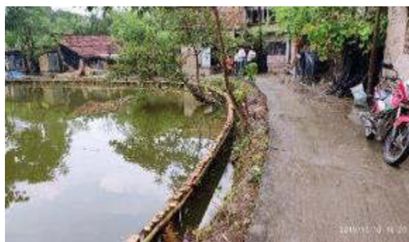
Bamboo piling before pipe laying seen at zone -9 (Pipe line)
