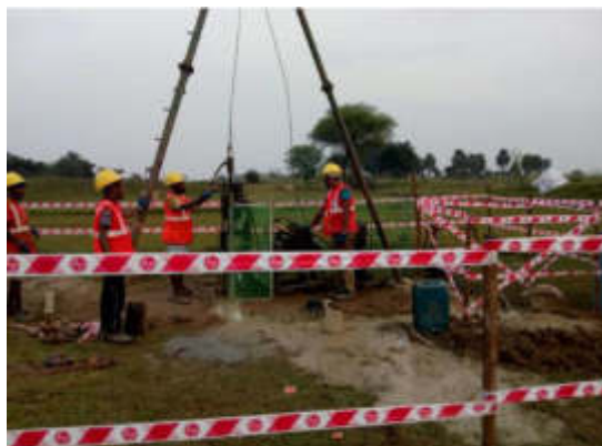
Geotechnical Investigation at Chakaltor OHR site
