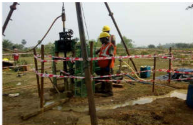
Geotechnical Investigation at Nayekhir OHR site
